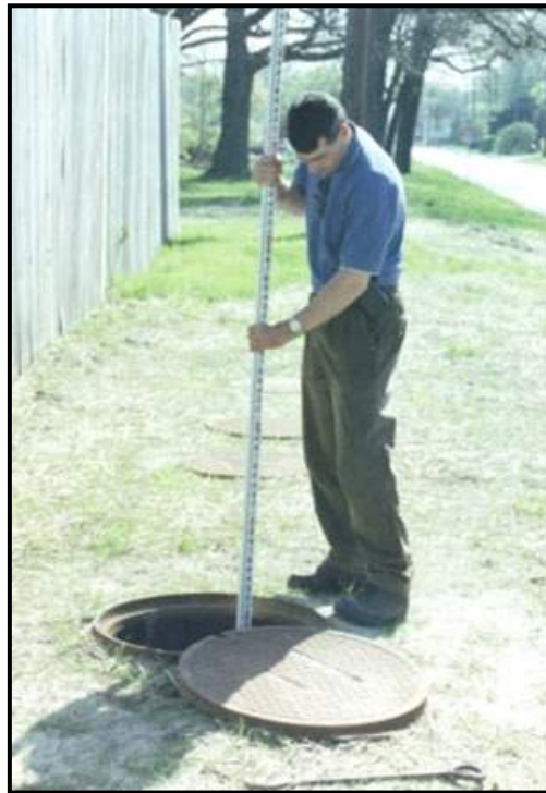
Sediment inspection using a stadia rod
