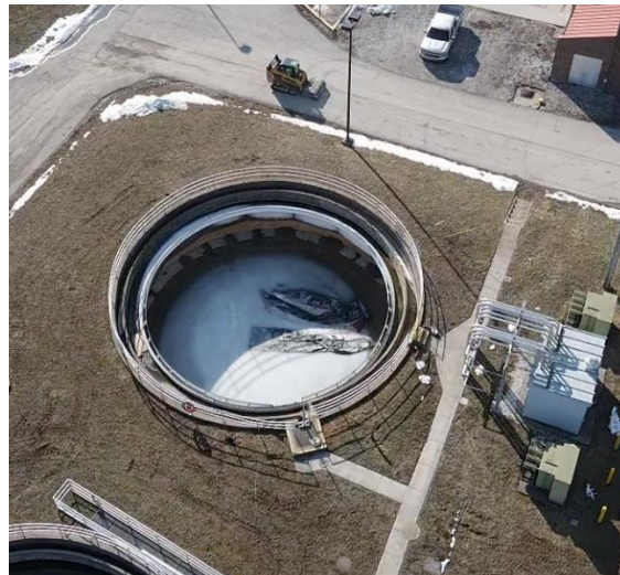
Clarifier equipment removed
