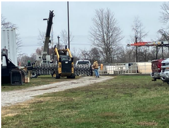
Rotor brushes going into ditch
