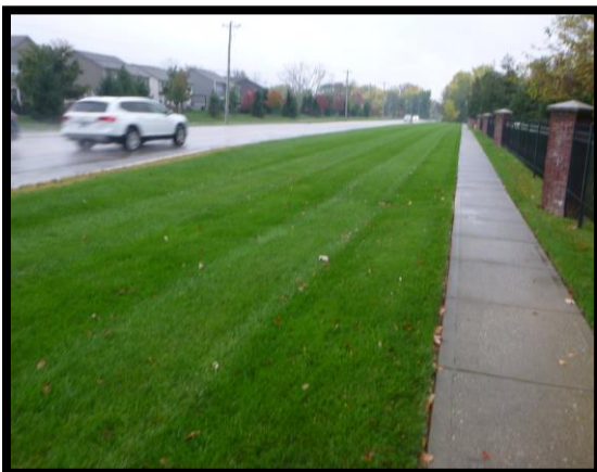
View of the roadside swale along CR 600 E, facing south.
