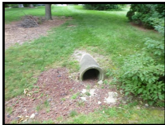
View of 18-inch RCP pipe that drains to the retention pond.
