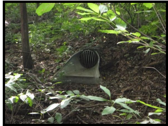
View of culvert pipe that runs under the B&O Trail.
